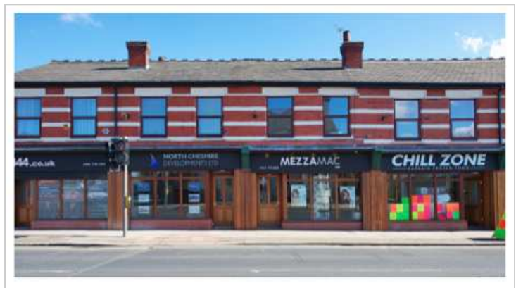
Above: The same shops have been refurbished as a block to ensure a unity of appearance. Individual shop fronts are separated by pilasters whilst signage allows individuality.
