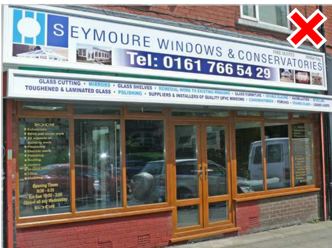
Above: Utilising a range of non-complementary materials and colours gives a fragmented appearance to shop fronts.
